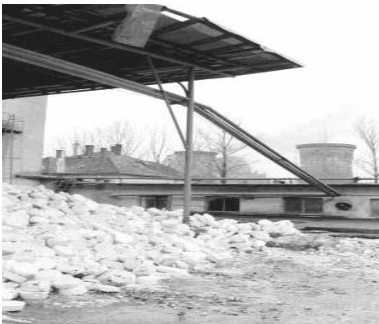
Figure 23.3. Storage of solids
